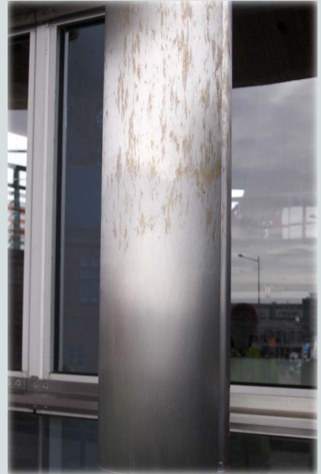
This column showed signs of corrosion shortly after installation. The lower area has been treated with Cleaner 61.
